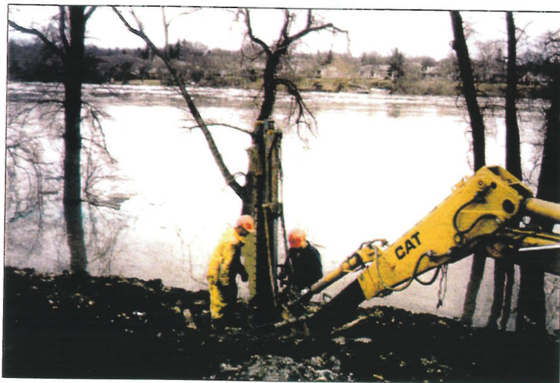
PHOTOGRAPH 4: VIEW OF DRILL RIG WHILE DRILLING BH01-48.
