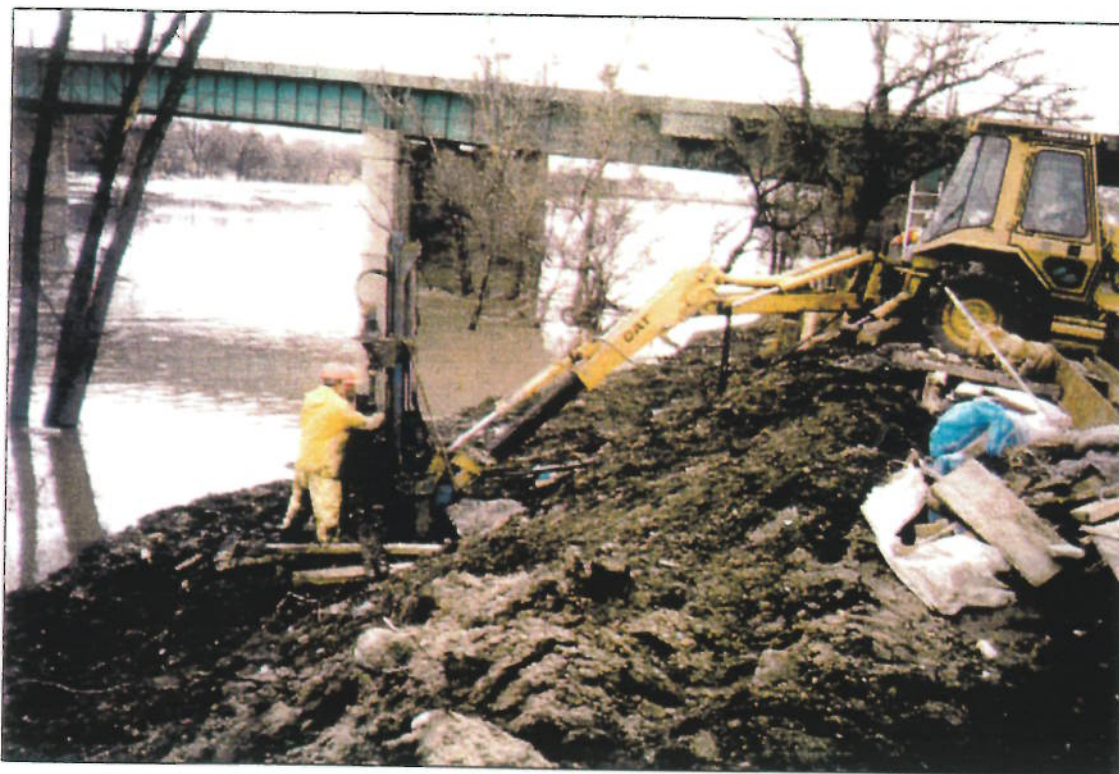
PHOTOGRAPH 3: VIEW OF THE DRILL RIG WHILE DRILLING BH01-47. GATE CONTROL STRUCTURE IS IN THE BACKGROUND (BEHIND BACKHOE).
