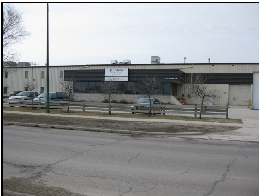
Photo 2 – Light industrial building located south of the Site.
