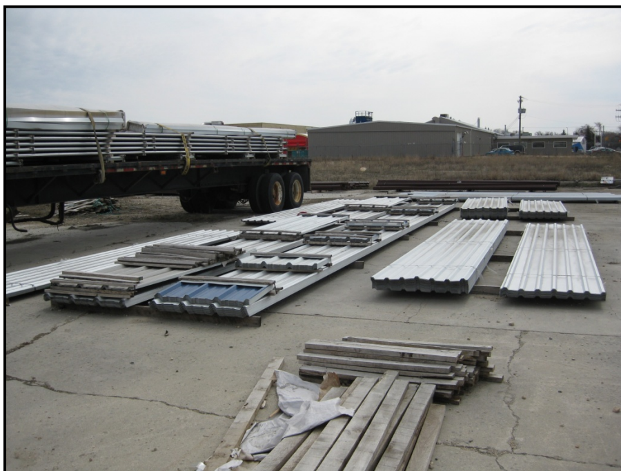
Photo 6 – Building materials stored on the southeast portion of the Site
