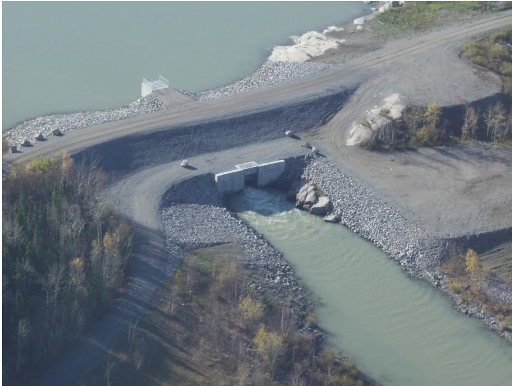
Photograph 6: Kiskitto Lake Inlet Control Structure (2004)
