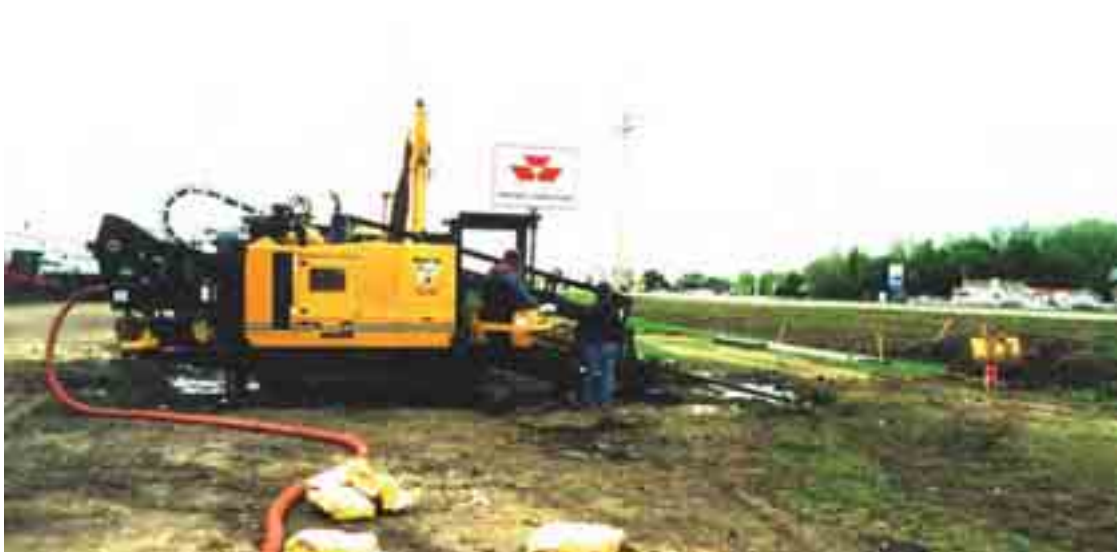
Pipeline is tunnelled under highway.
