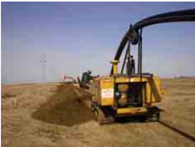
Trencher installs pipeline.
