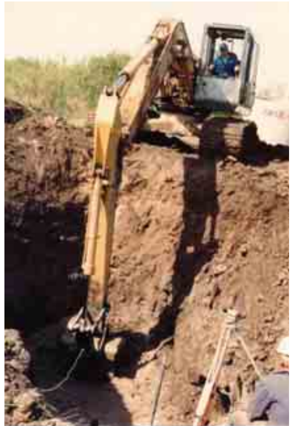
Backhoe installs wet well
