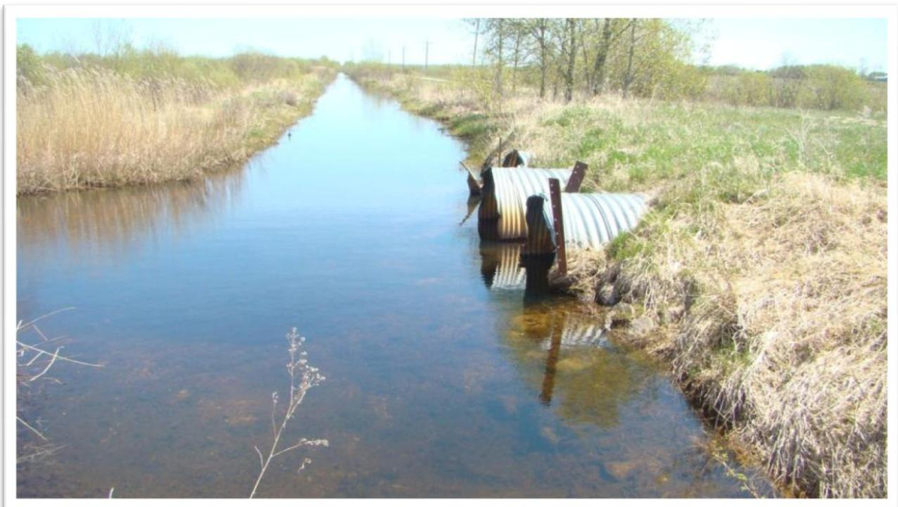
**Figure 14:** Existing culverts at the old PR 201 crossing
