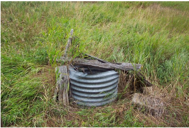
An improperly sealed well in the West Souris Watershed. Source water protection will be one component of the integrated watershed management plan.
