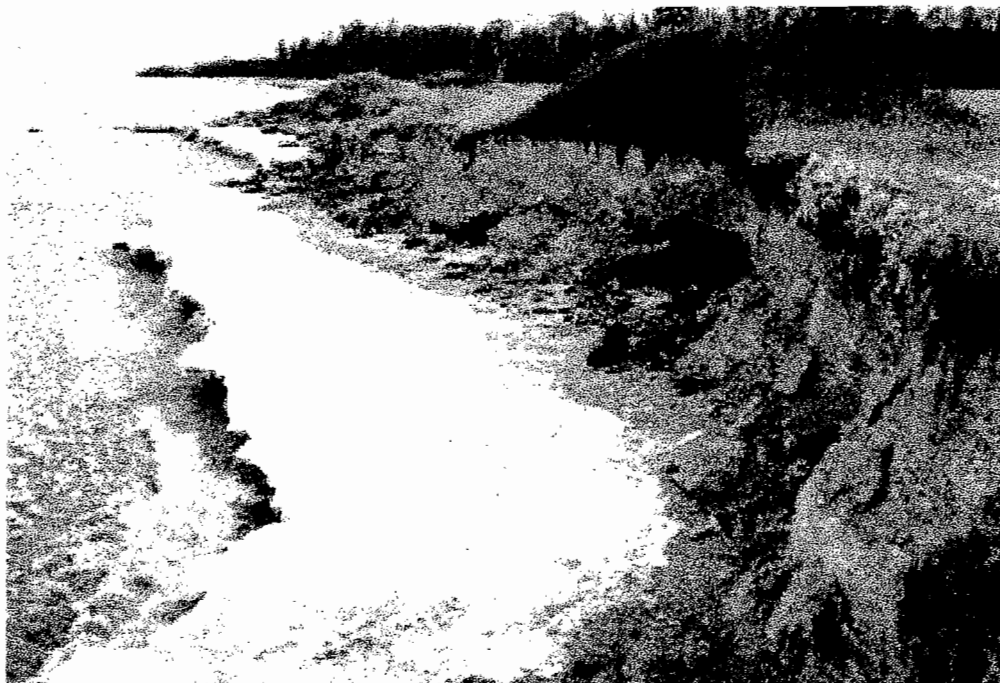
Figure 19. Eroding cliffs north of the town of Gimli. View looking south.
