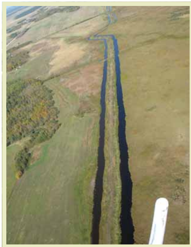
Aerial view of a drain in Washow Bay area | Figure 15.
