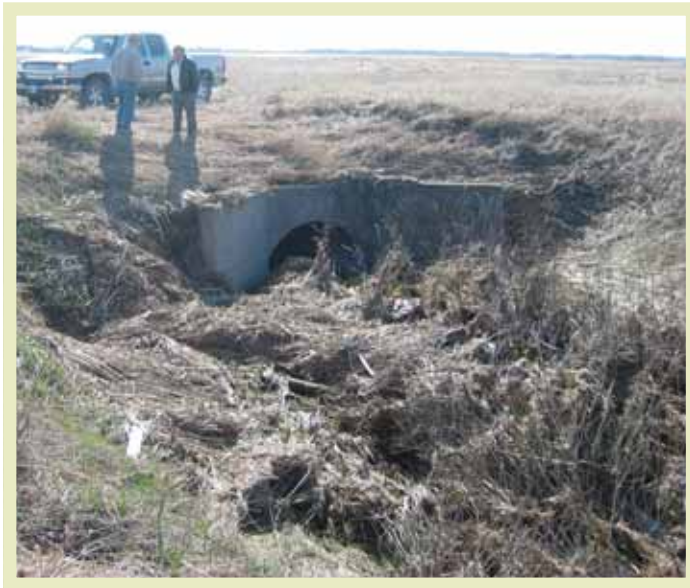
An overgrown drain in the Icelandic River and Washow Bay Creek watershed. | Figure 16.
