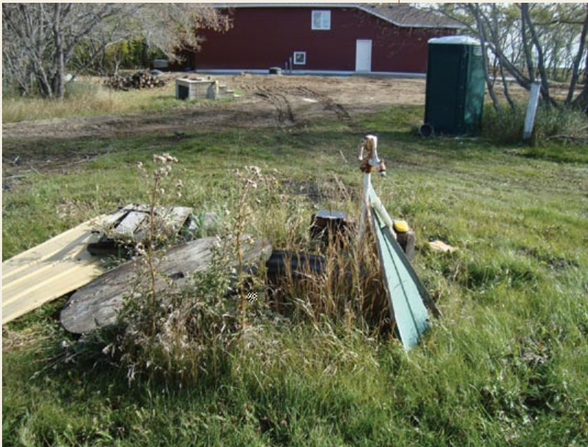
Figure 11 - Old, abandoned, or poorly maintained wells such as the one pictured below represent a potential threat to groundwater aquifers.
