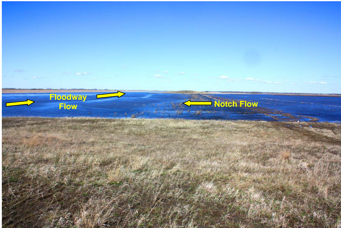
Figure 3: Flow through the west notch on May 2 nd , 2011.
