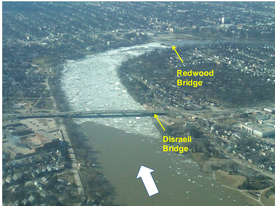
Figure 2: Ice jam between Disraeli and Redwood Bridges on April 7 th , 2011.
